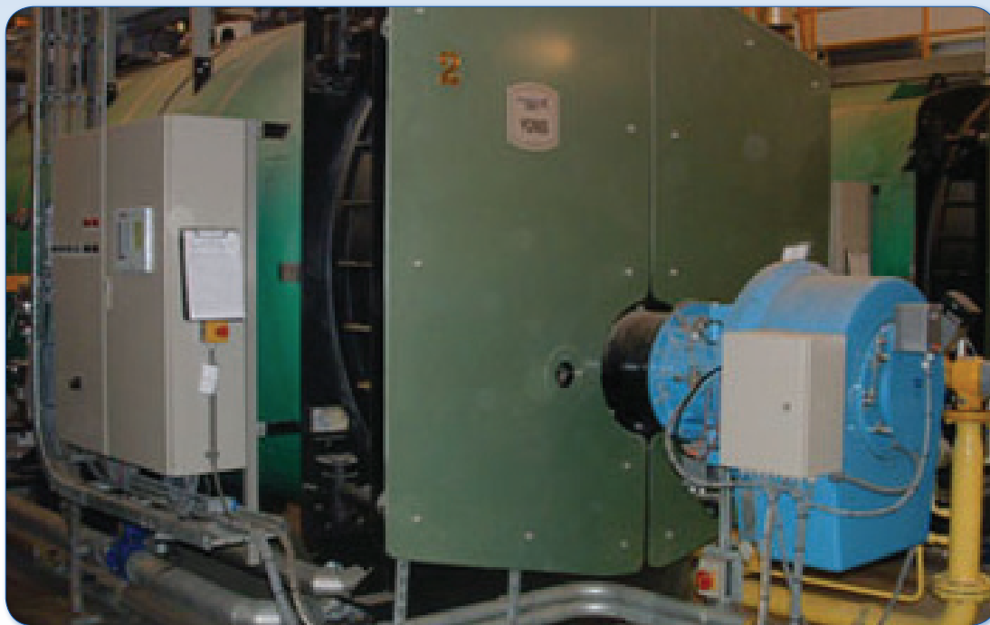
Above: New Burner Management Controls
