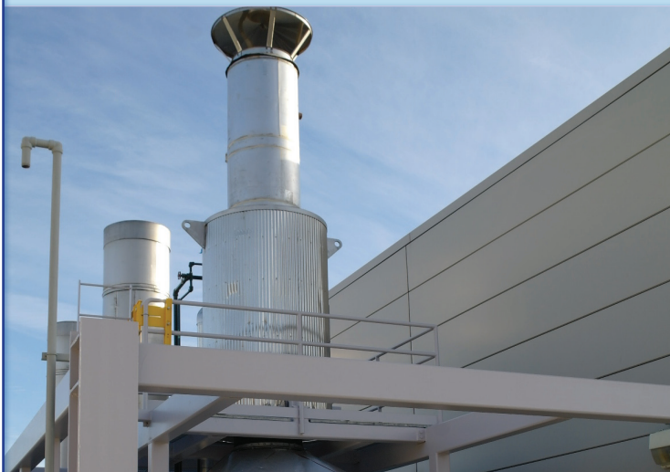
Above: Induced FGR for low NO x Below: Low Emissions Exhaust Stack
