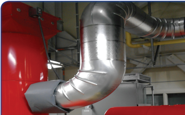
Above: Induced FGR for low NO x Below: Low Emissions Exhaust Stack
