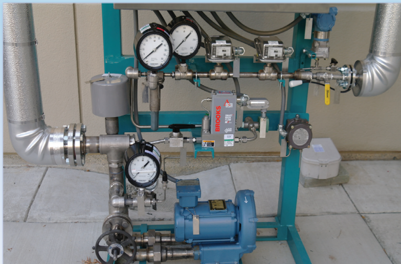
Above: New Limpfield burners. Below: NO x Reducing System
