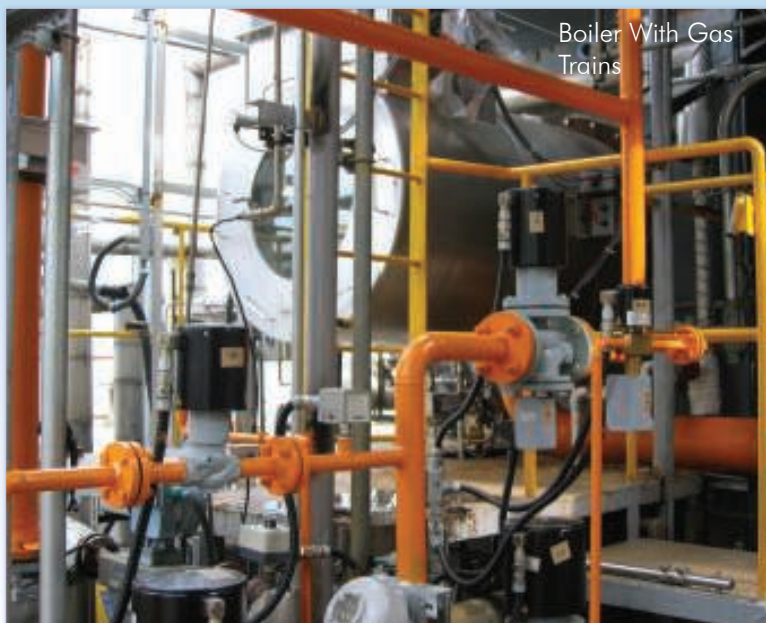
Above: 25 Tonne Boiler Installed
