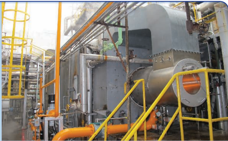
Above: 25 Tonne Boiler Installed
