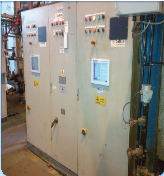
Panel Retrofitted With Mk7 Controllers
