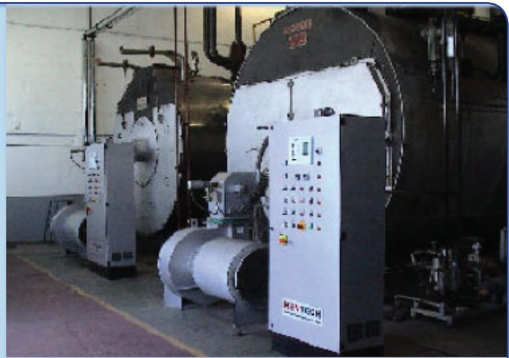
Above : 2 Boilers with Autoflame and Pressure Jet
